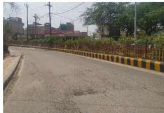
Dense plantation in median causing vision obstruction
