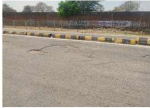
Sufficient paved shoulder not available throughout the stretch.
