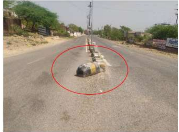
Curb stone in travel lane is serious safety hazard.
