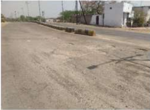
Sufficient paved shoulder not available throughout the stretch.
