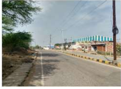
Sufficient paved shoulder not available throughout the stretch.
