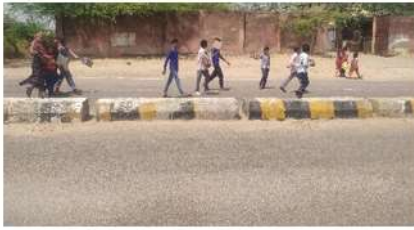
No traffic calming measures available at locations of frequent pedestrian crossings.
