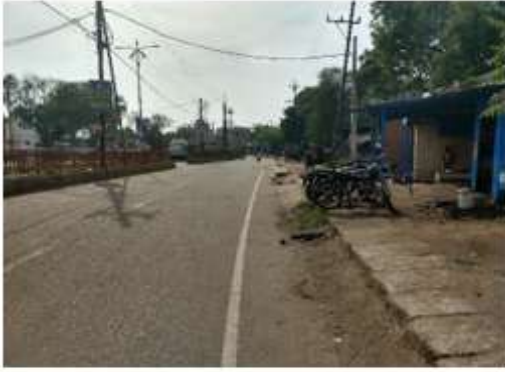
Sufficient paved shoulder not available throughout the stretch.
