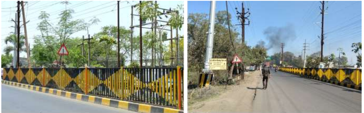
Only two traffic signs are observed throughout the stretch
