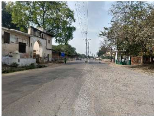
No Signage for the intersection.
