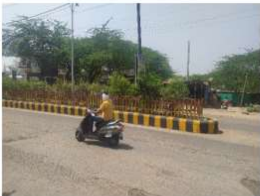
Dense plantation in median causing vision obstruction
