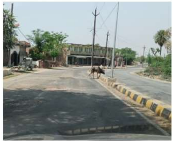
Curb stone in travel lane is serious safety hazard.
