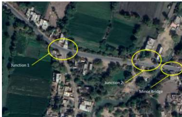
Figure 20: Satellite Image of the Blackspot at Tawai Bujurg
