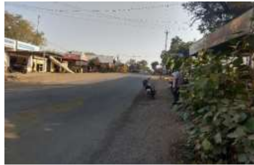
South approach of the junction
