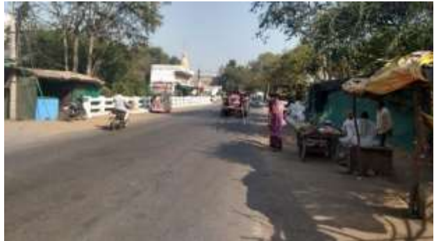
Bridge south of Junction 2
