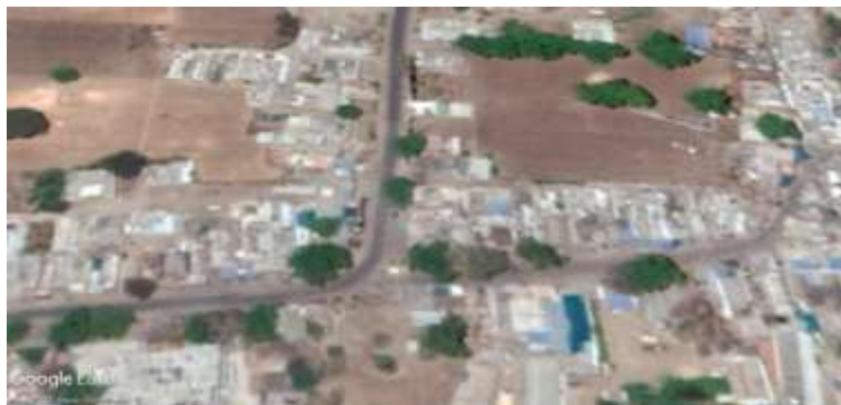
Figure 24: Satellite Image of the Bakaner Junction
